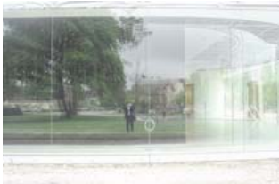
Exterior's detail Photograph
