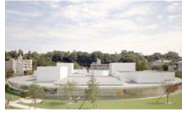
Sight of the exterior Photograph
